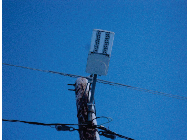
LED Street Light Installation
