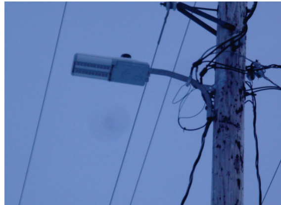
LED Street Light Installation – Second View
