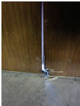
Mechanical Room Doors
