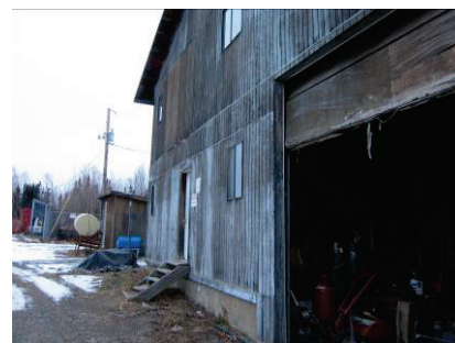
Building Exterior and Overhead Door
